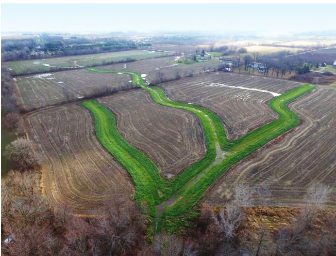
Grassed waterway in Silver Creek: before and after installation.
